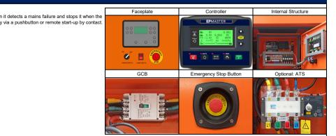
Protection, distribution, and automatic control panel, which starts the generator set when it detects a mains failure and stops it when the mains is restored with the control unit EPM4. It also starts and stops the group manually via a pushbutton or remote start-up by contact.
